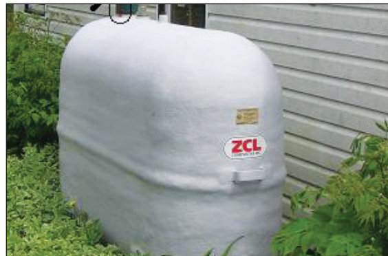
Sample of Fiberglass Tanks
